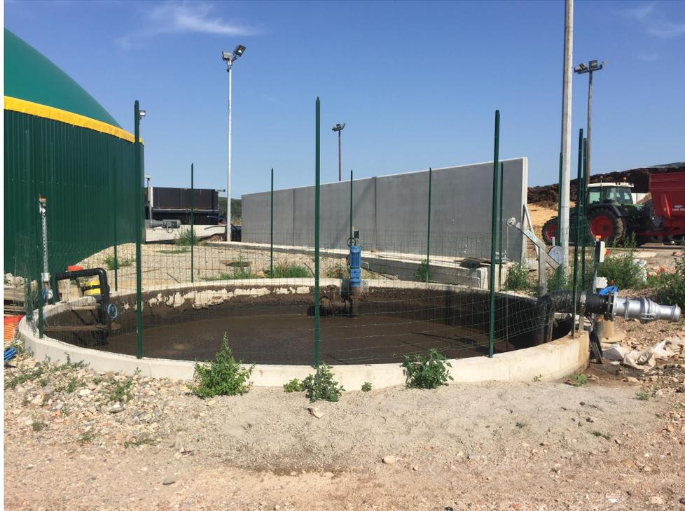
**FIGURE 8 : LA PRÉFOSSE D'INCORPORATION DES SUBSTRATS LIQUIDES**
